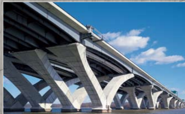
Woodrow Wilson Bridge, Washington, USA
